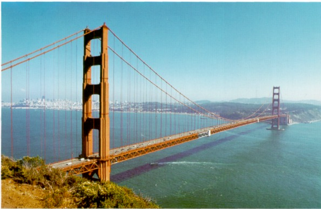
14.12 - Golden Gate Bridge with San Francisco in the background.
